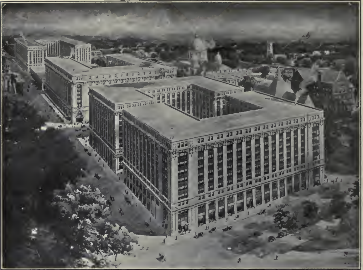
The Montreal Terminal Station for the Canadian Northern Railway, now in course of erection.
